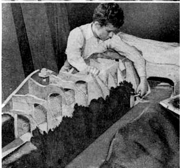
Fig. 25. Wire mesh is next tacked or stapled over the form. Do not pull it taut, but allow slack so it can be shaped and bent between the forms to make gullies and ravines. Material troweled on wire is mixture of brown plaster and asbestos.
