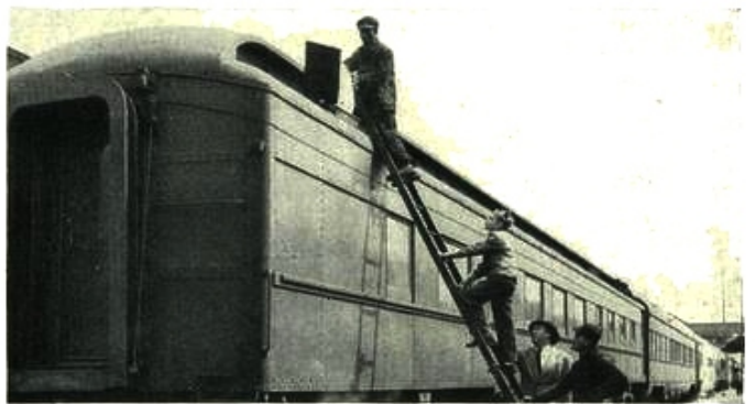
Because dining cars carry so many perishable food items, the big refrigerators must be kept chilled. Here an employe of the passenger car yard has opened a bunker door above the dining car kitchen and is about ready to let a hundred pound piece of ice slide down into the box.
